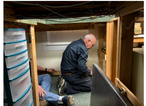
Installing some shelves in the Lionel Room
