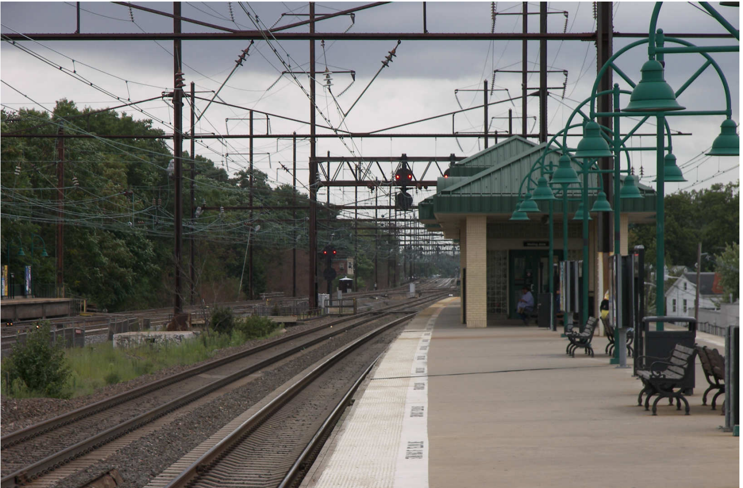
Above: On the platform, looking south. The old Pennsy position light signals are still in use, but have been recently relamped for 2 colored lights instead of three amber. Union Tower, beyond, still protects Union Interlocking, the junction of the Northeast Corridor and the North Jersey Coast Line. Below left: Amtrak Metroliner control cab 9638 leads a rare consist pushed by an AEM-7. Lower right: NJ Transit ALP-46 No. 4601 pauses it's train of bi-levels on Track 6 on its way to the Amboys and Bay Head. NJ Transit operates its trains push-pull fashion, typically with locomotives leading outbound from Penn Station. Today, though, many trains seem to deviate from this norm.
